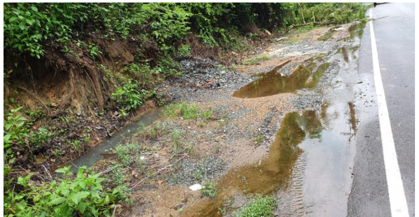
Fig No.1.Critical Area of Drain (i)
