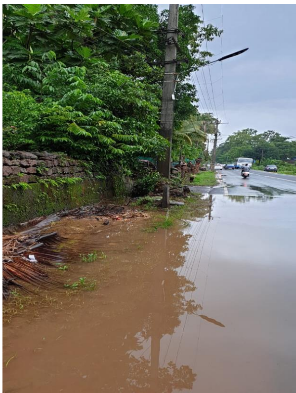
Fig No. 3 Water Entering on Road
