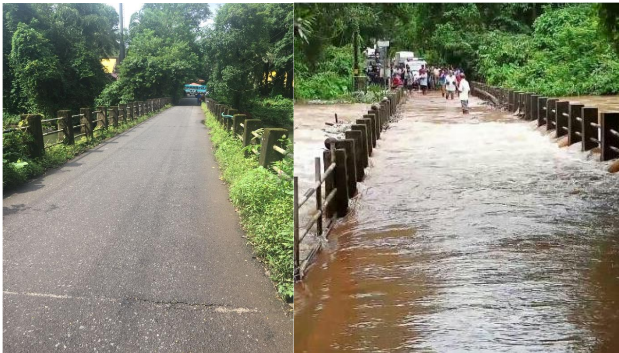
Fig1 Bridge during dry season
